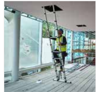
Shown fully deployed accessing a ceiling void
