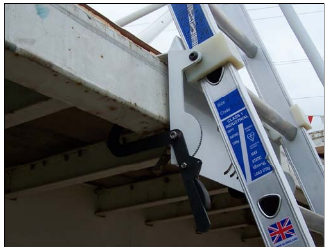
Figure 2 Showing ratchet clamping system
